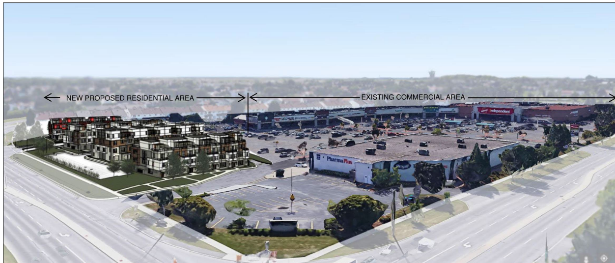
Figure 2. View from the North West corner of the site – Corner of Jeanne D'Arc Blvd. and Orleans Blvd.
