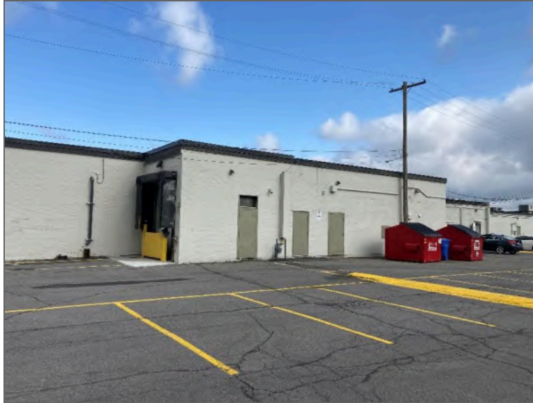
Photo 3 – Site Building (southeast elevation).
