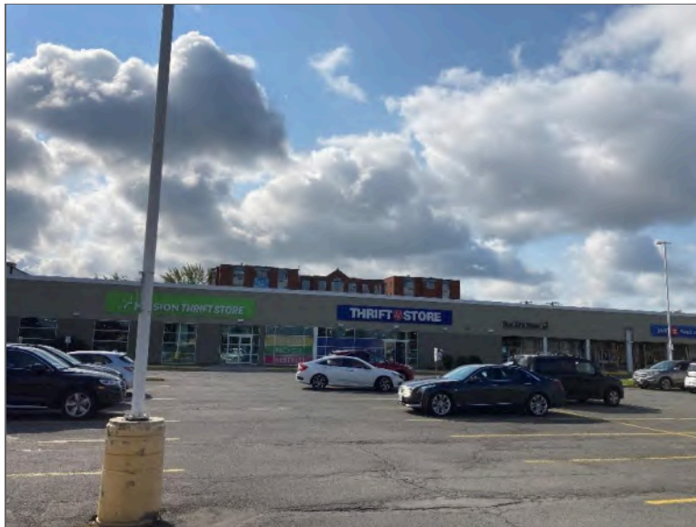
Photo 4 – Site Building (southwest elevation).
