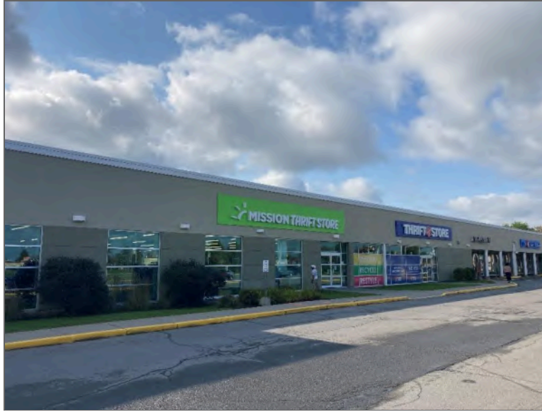
Photo 1 – Site Building (northwest elevation).
