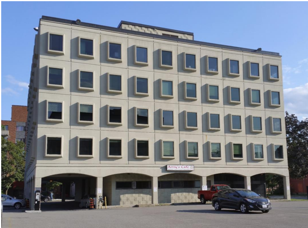
Figure 10: The view looking south towards the low rise building from the parking lot with the arcaded auto-oriented drop-off entrance at the parking lot side of the building. The style of this 4-square is described in the ERA evaluation sheet as a Brutalist Post-modernist vernacular low-rise commercial office building.
