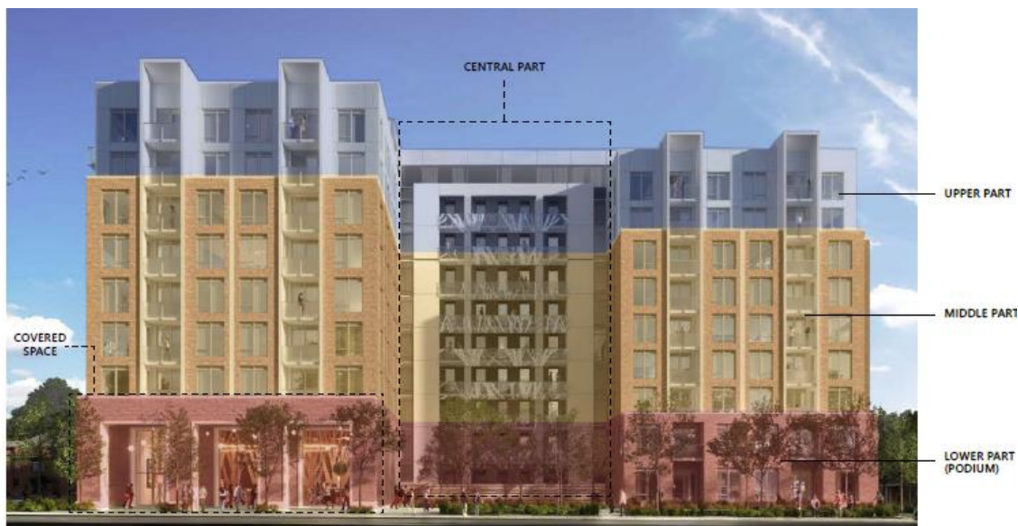
Figure 15: Contextual analysis and the building’s massing, rhythm, and vertical organization. Source: Neuf Architecture 2023.
