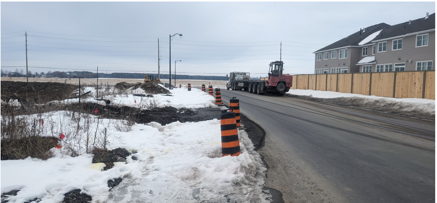
Photo 2 - Facing northeast towards the intersection of Cosanti Drive and Shea Road. The Site is to the left and the residential dwellings (located along Maverick Crescent) are to the right.
