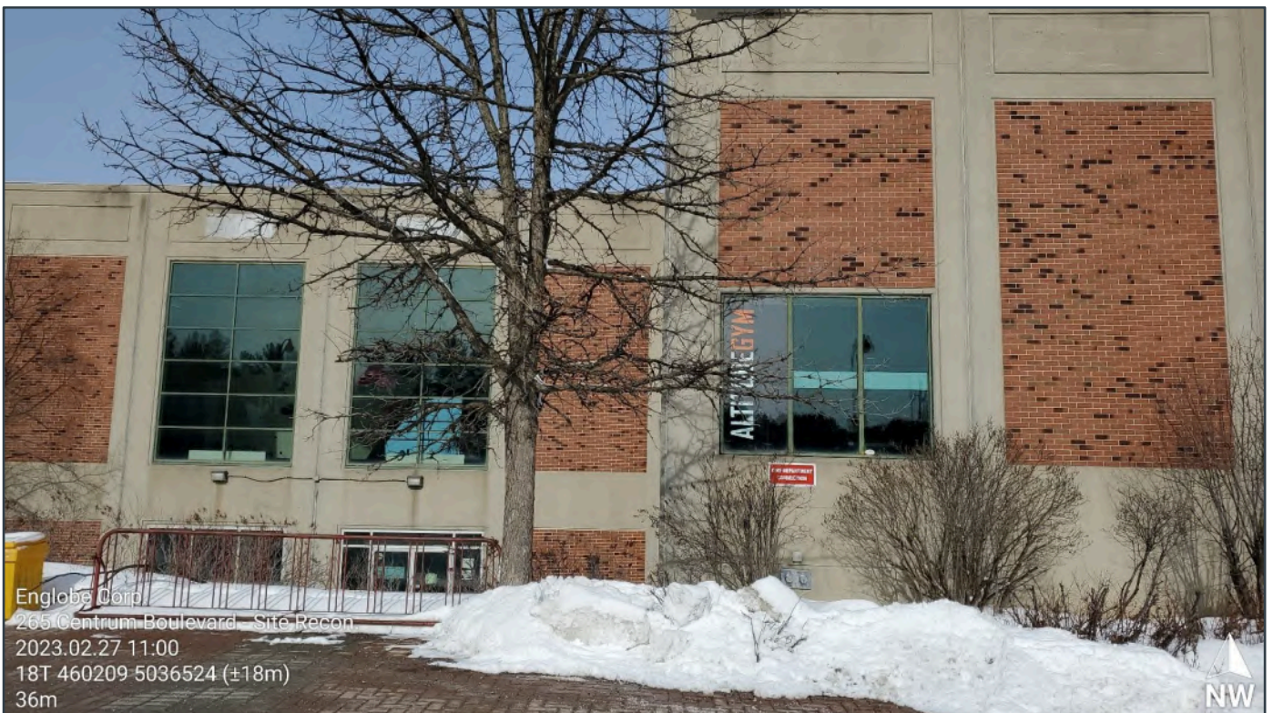
Site Photograph 2: Overview of the Site building (original build).
