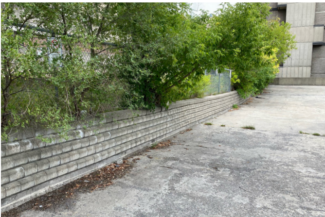
Retaining wall and grade change at south site boundary.
