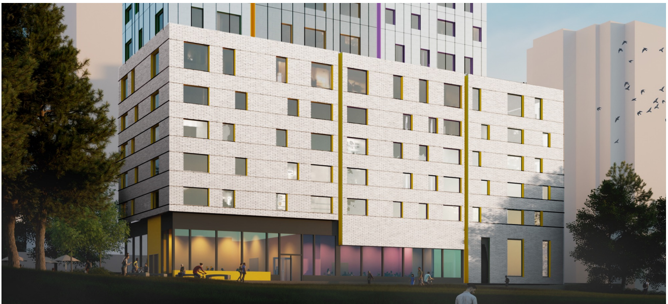
Overall view of building podium.
