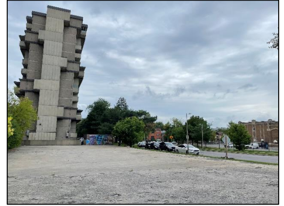
Figure 2-6: Site, looking west towards existing underground parking garage at 200 Friel Street
