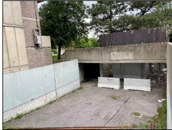
Figure 2-11: Entrance to existing underground parking garage on site
