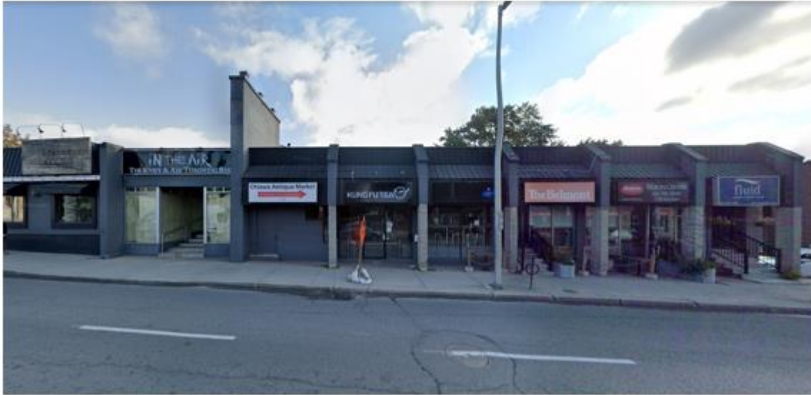
7 BANK ST, LOWRISE COMMERCIAL VIEW FROM PROPERTY – WEST
