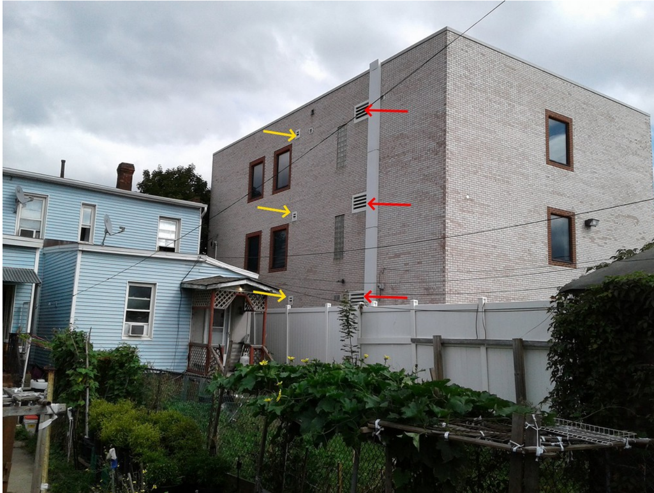
Figure 3: View of the North Facade of the Embassy of Madagascar
