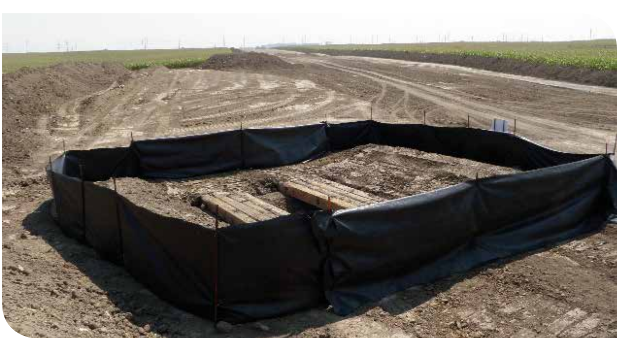
Cleaning station at construction site.
