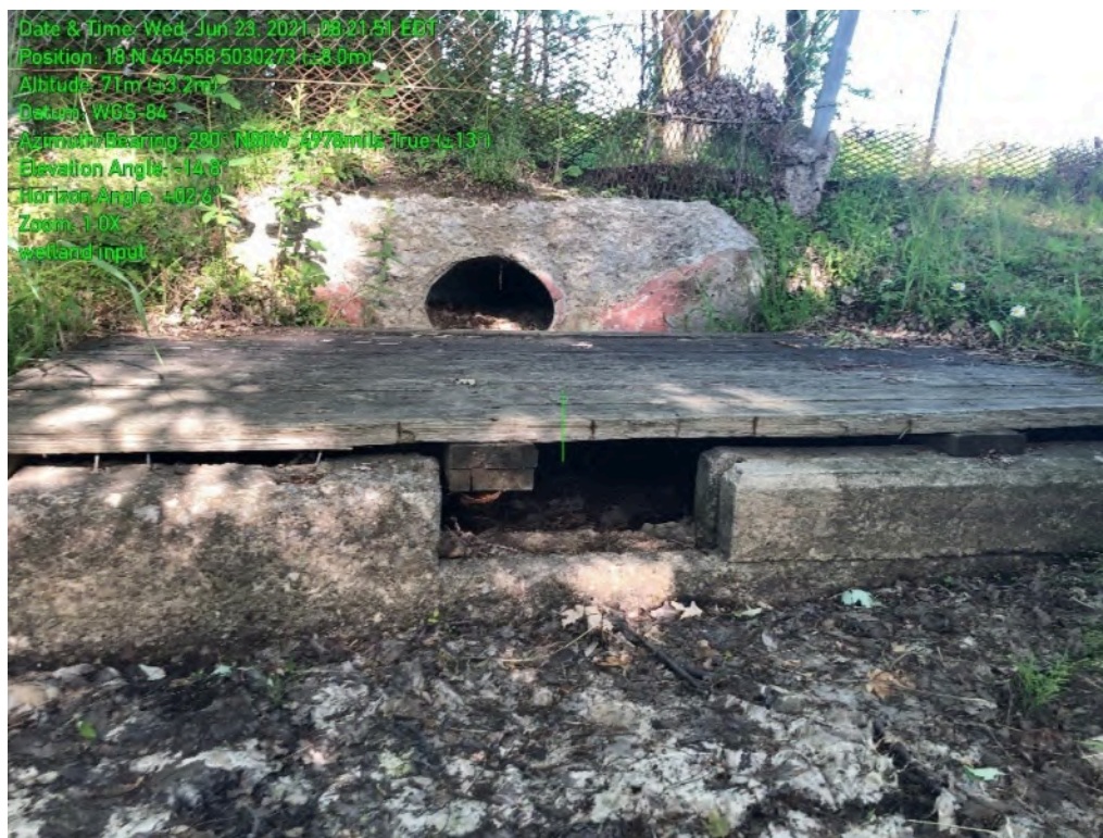
Figure 8 Photo showing the remnants of a dike in the northwestern portion of the wetland on Site (taken June 23, 2021)
