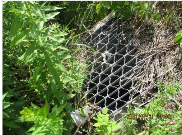
P2 – Ditch inlet at Innes Road
