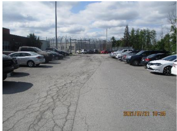
P4 – Fire Route (looking south)
