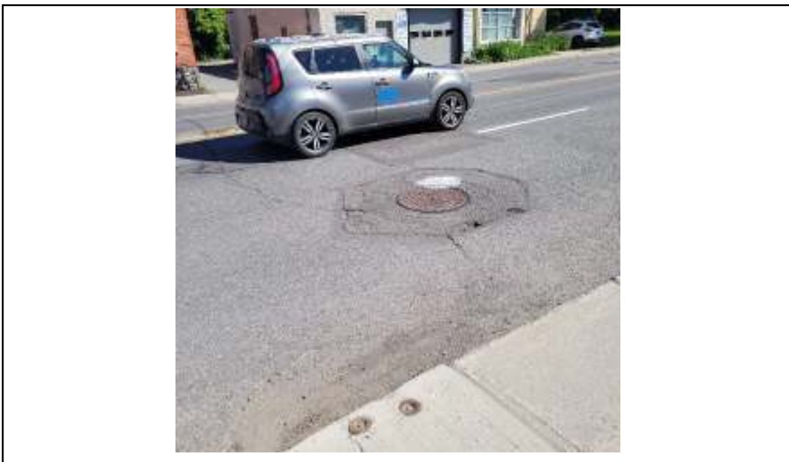
Photograph 26: Storm water manhole on Hawthorne Avenue, water service valves in sidewalk in front of 20 Hawthorne with former automotive service center across street at 25 Hawthorne.
