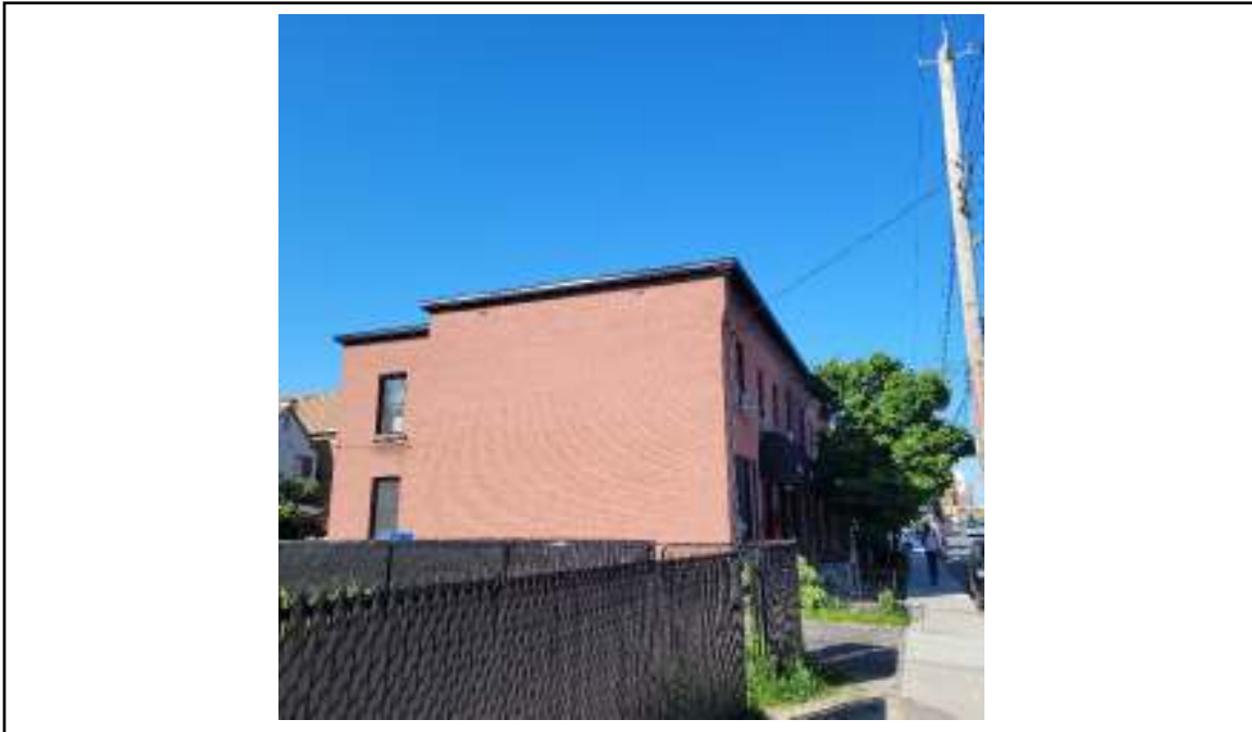
Photograph 3: Looking west from sidewalk of 20 Hawthorne towards buildings at 12-18 Hawthorne.
