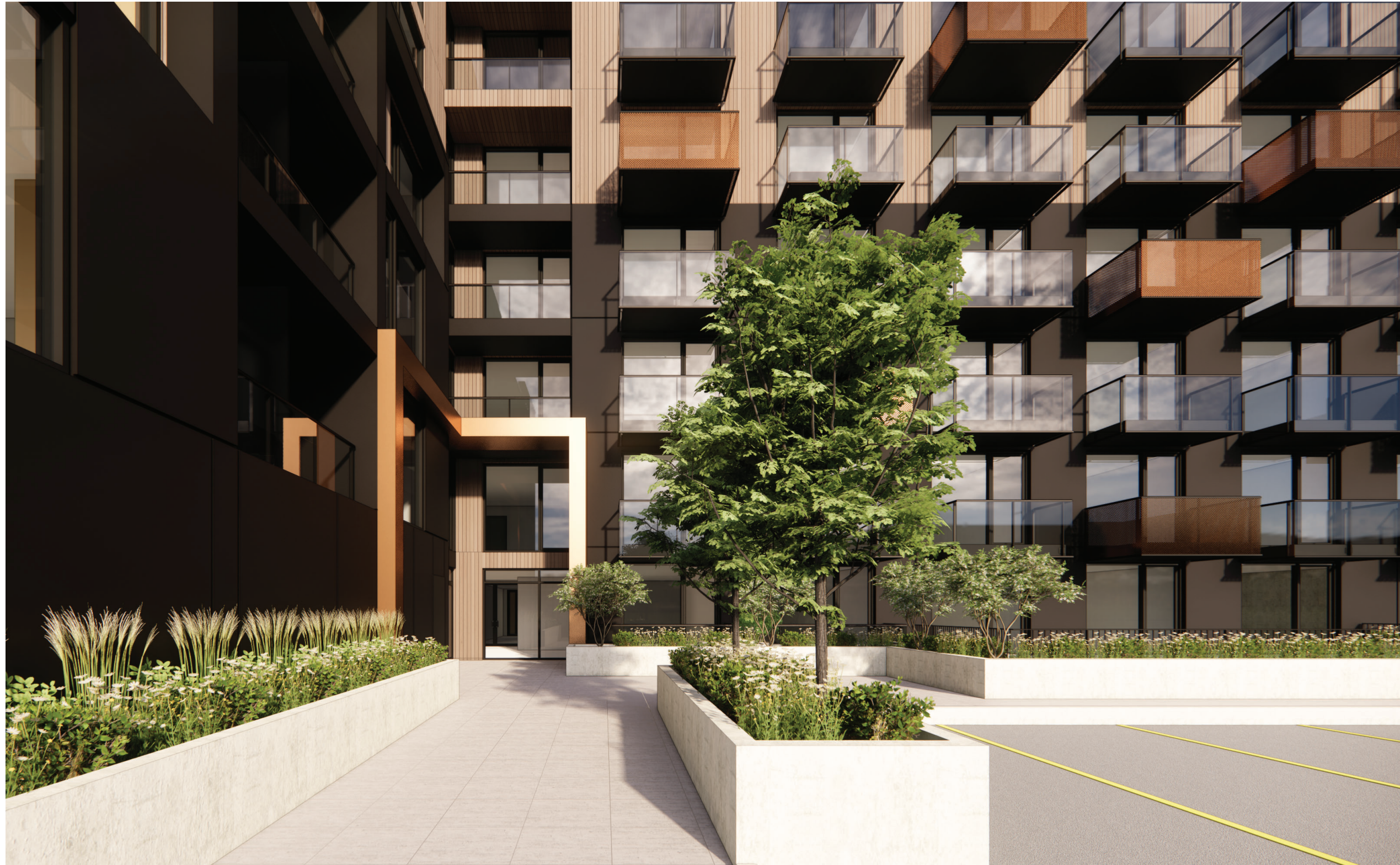
View of Rear Entry
