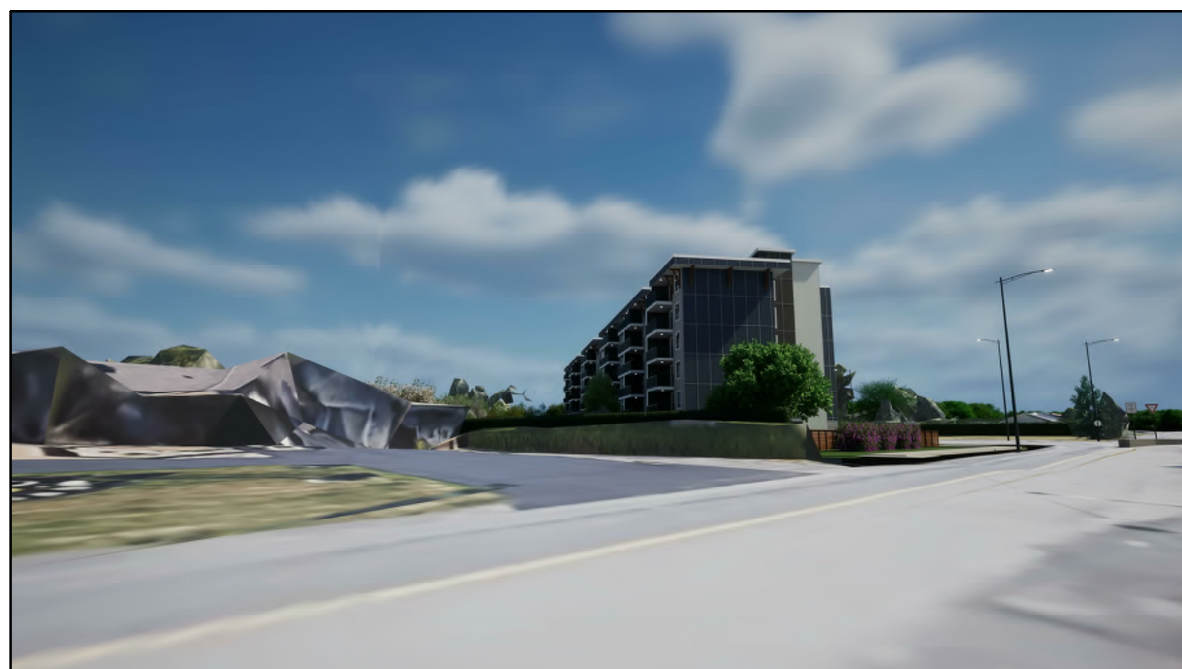
(3) NORTH - WEST VIEW
