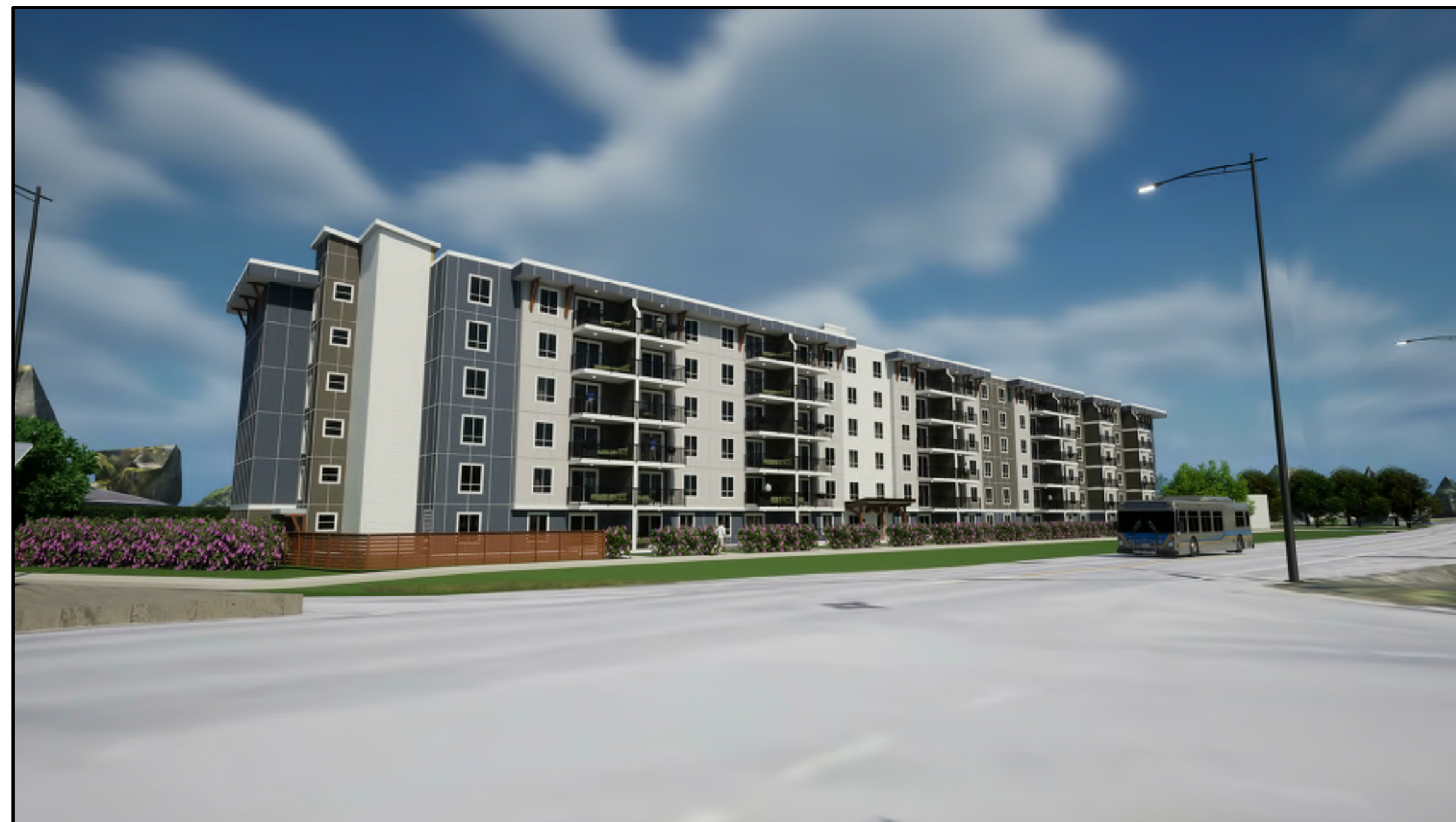
(1) SOUTH - WEST VIEW
