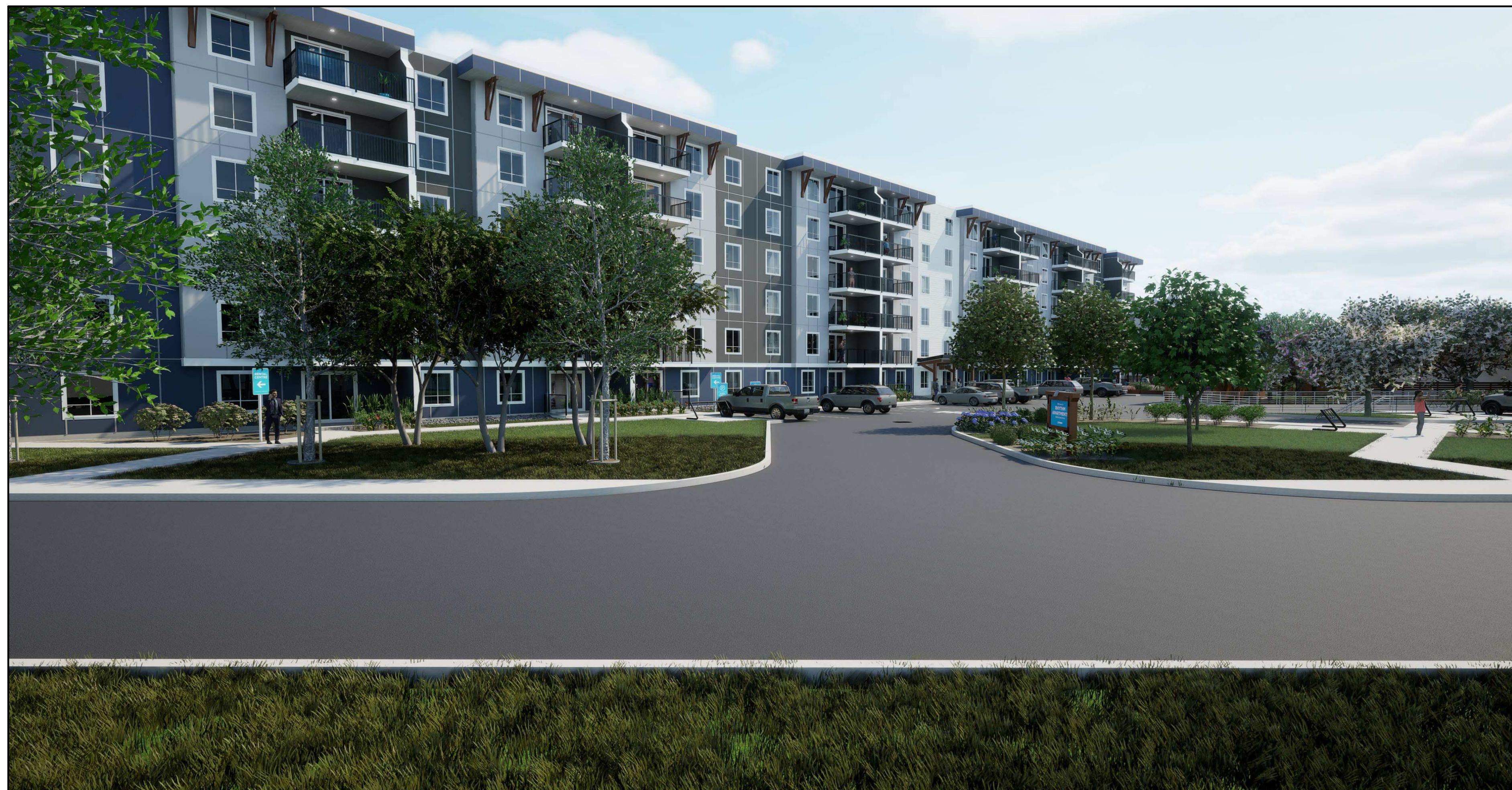
(2) EAST VIEW SITE ENTRANCE
