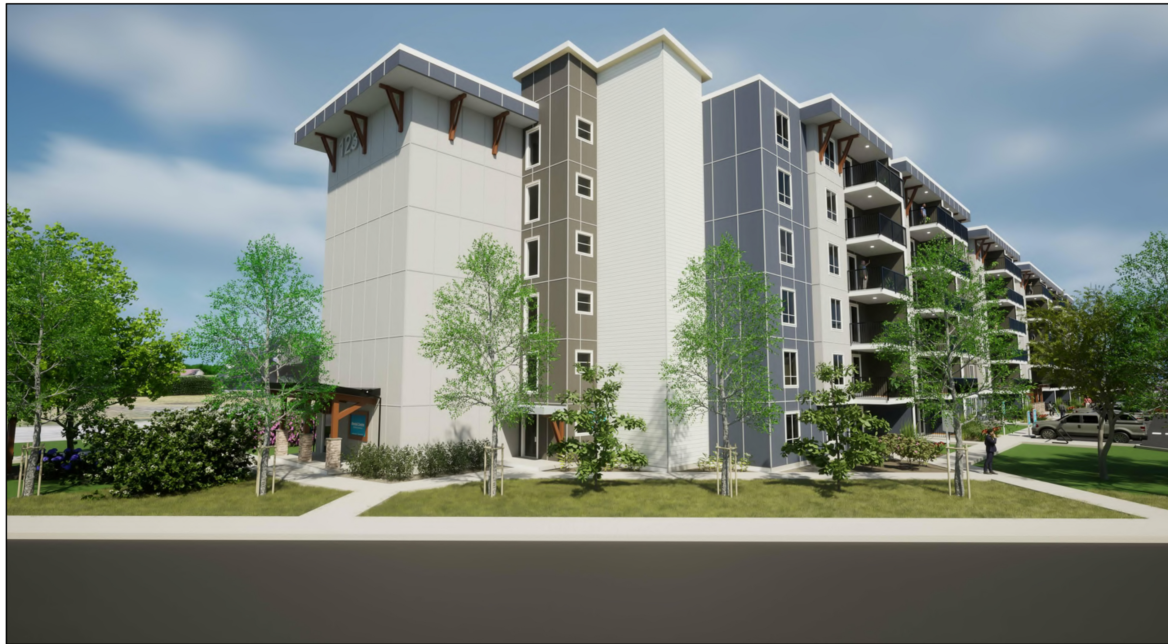
(1) EAST VIEW BUILDING CORNER ENTRANCE
