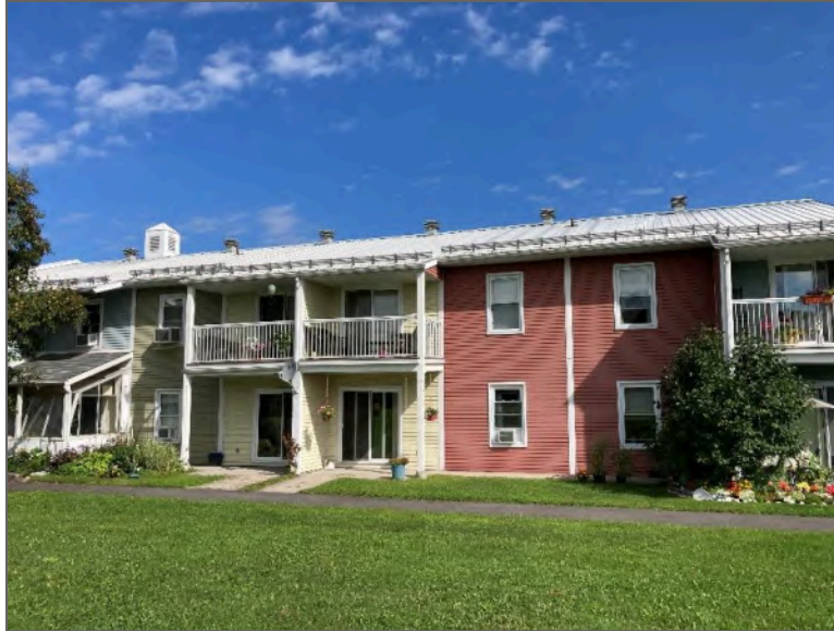
Photo 3 – Site Building (south elevation).
