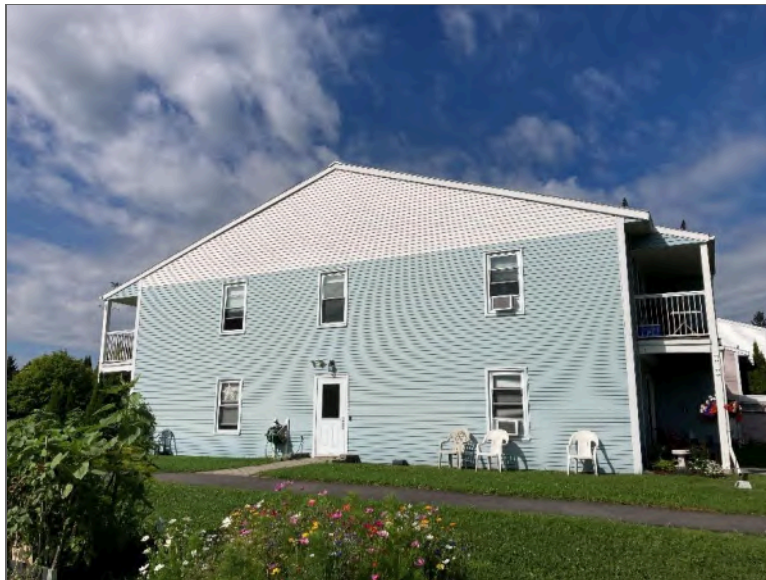
Photo 2 – Site Building (east elevation).
