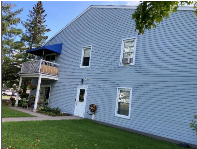
Photo 4 – Site Building (west elevation).
