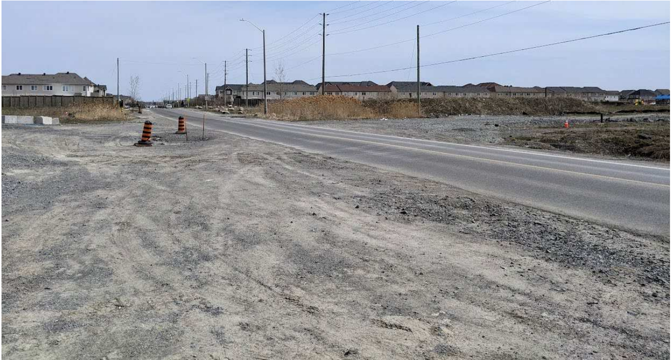
Figure 6: View of Cambrian Road, looking southeast from the site (Parsons, April 2023).
