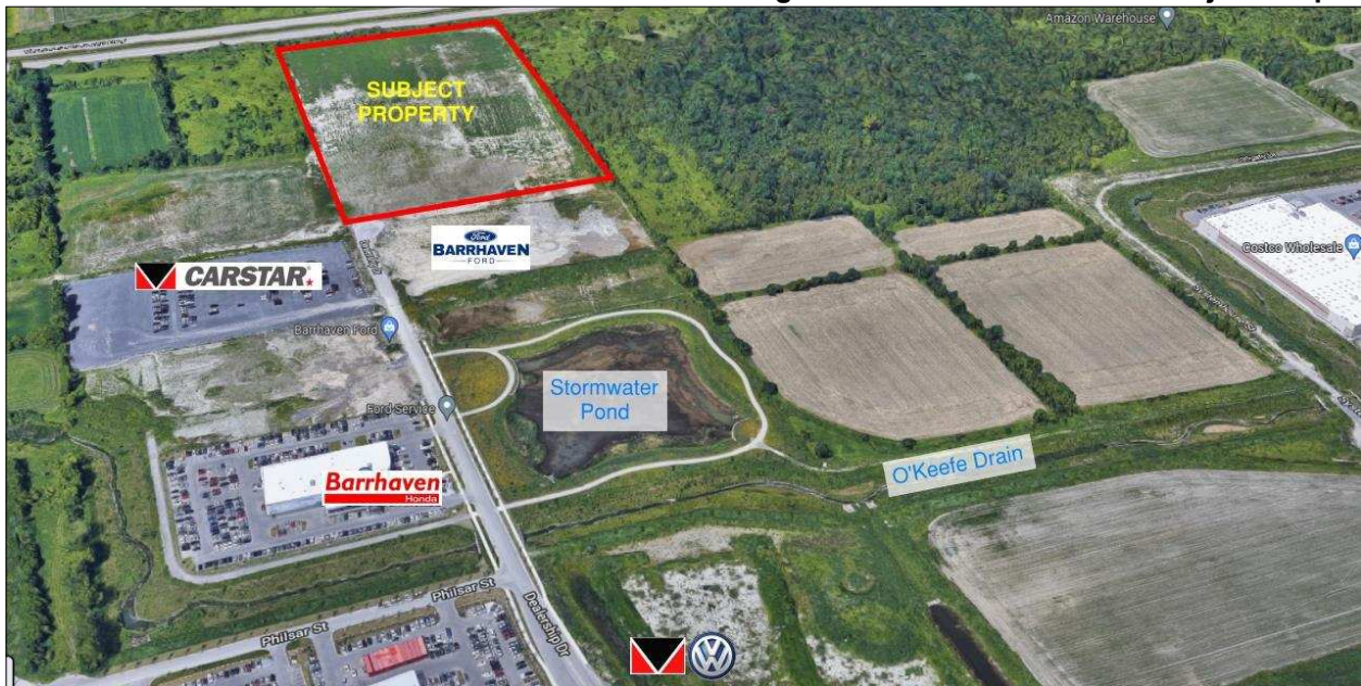
Figure 4 – Land Uses East of Subject Property
