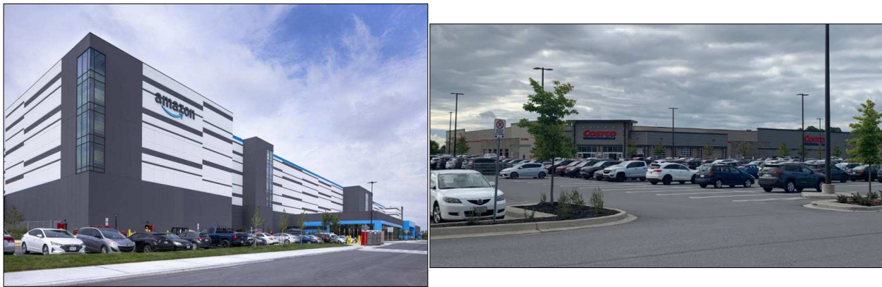
Figure 2 – Land Uses North of Subject Property
