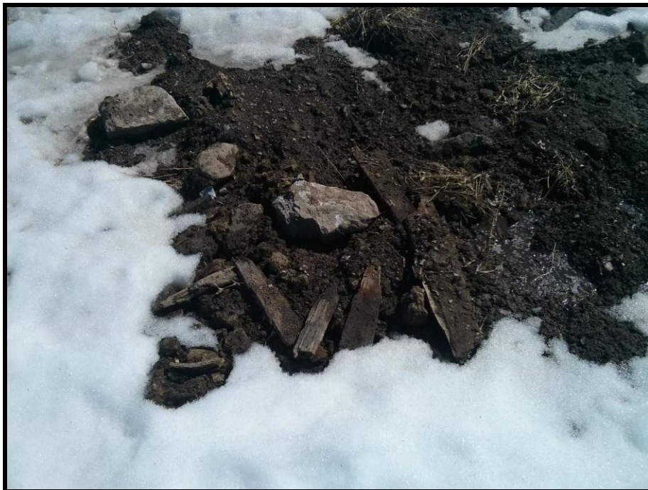
Photograph 6: View of recent soil disturbance from test pits (demolition debris present in the fill)
