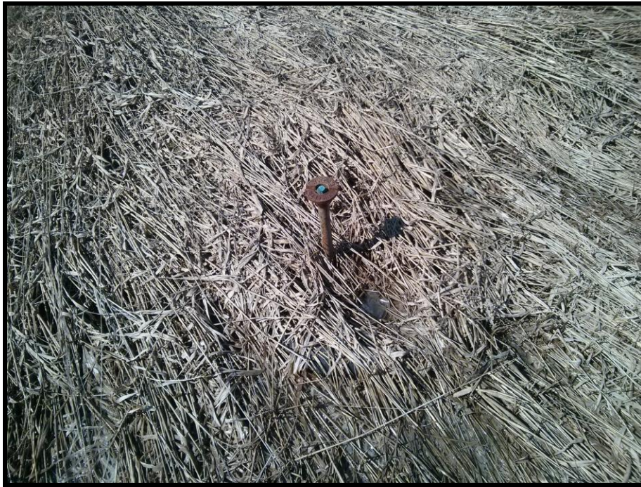
Photograph 3: View of a water shutoff valve located in the southwest corner of the site.
