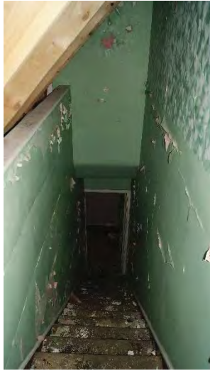
Stairs to basement
