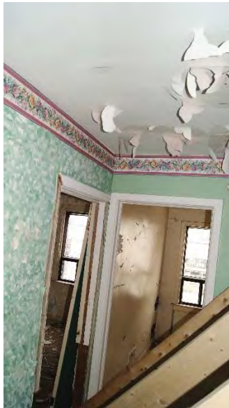
Second Floor (living room)
