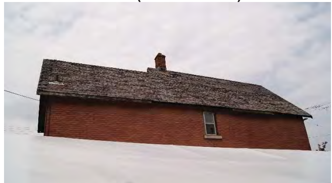
Roof (view from south)
