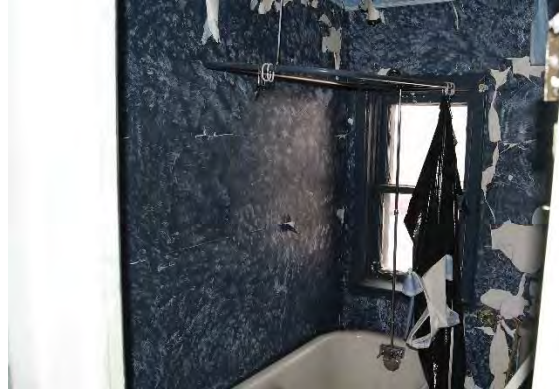
Second floor (bathroom)
