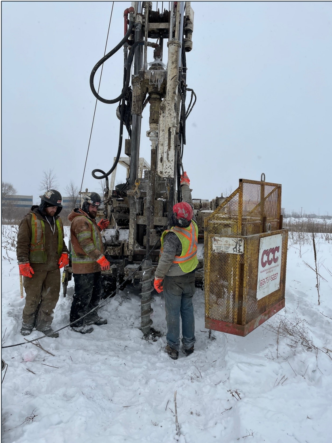
Site Photograph 1. Overview of drilling operations (February 21 to February 24, 2023).
