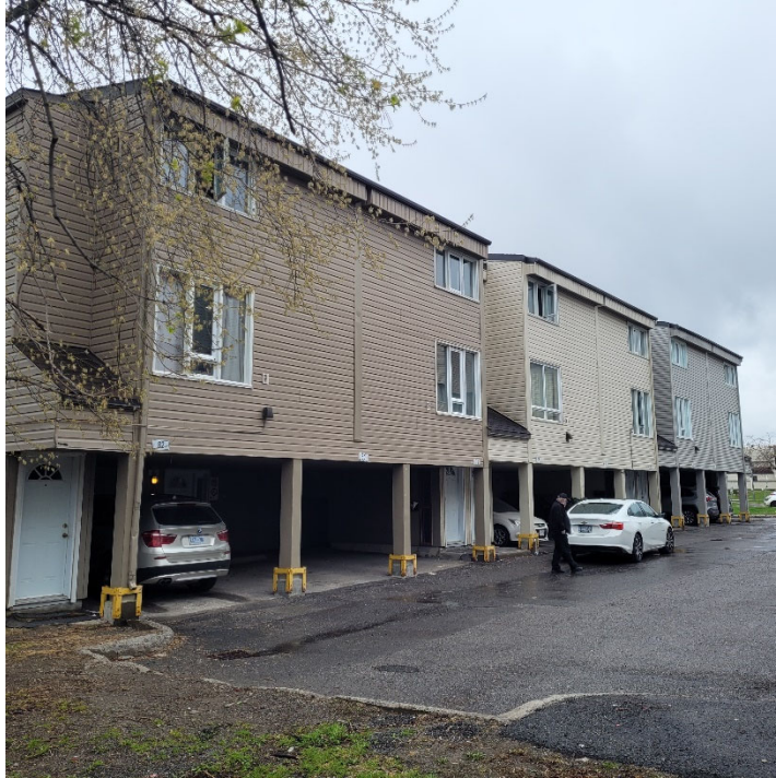
Photograph 3: View of residential building at the Phase One Property looking west-southwest from Finch Private (April 24, 2023).
