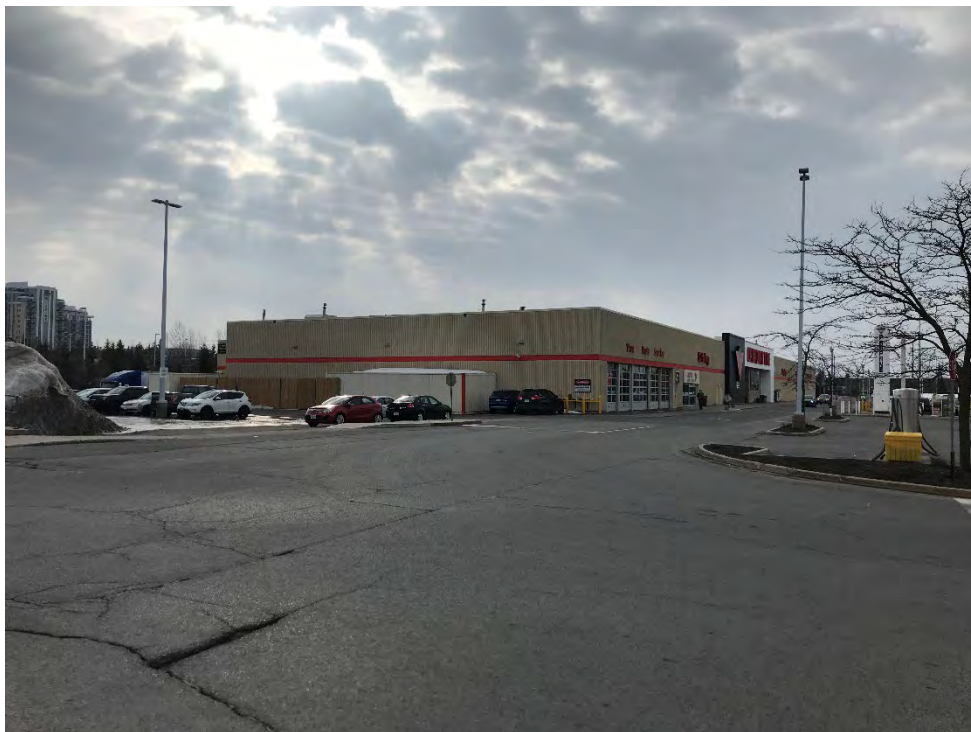
Photo 2 View of Automotive Service Centre at 2501 Greenbank Road, Ottawa, Ontario at the northern portion of the Site, facing southeast. March 29, 2023.
