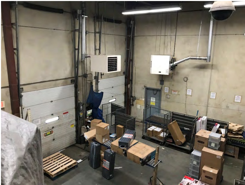
Photo 20 View of the loading area within the Warehouse in the Canadian Tire Retail Store. March 29, 2023.
