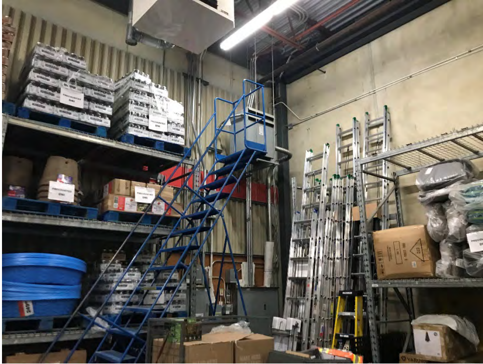
Photo 19 View of transformers located in the southeast corner of the Canadian Tire Warehouse. March 29, 2023.
