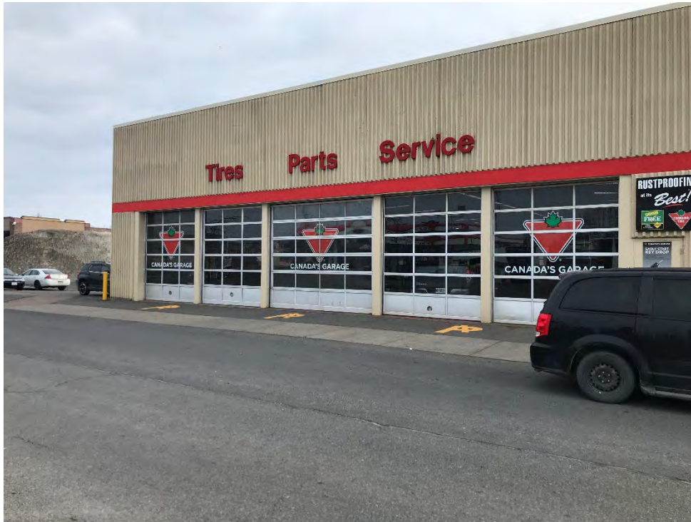
Photo 3 Outside view of the Automotive Service Centre, facing northeast. March 29, 2023.
