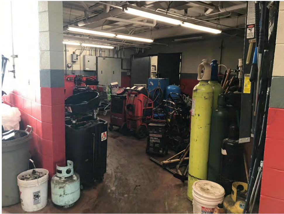
Photo 31 View of helium, oxygen, and Acetylene gas cannisters in the Automotive Service Centre. Staining on the floor is visible. March 29, 2023.
