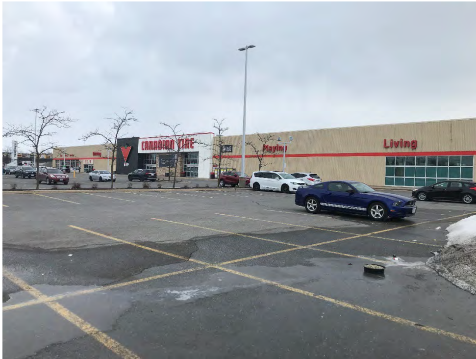
Photo 1 View of Canadian Tire Retail Store (CTR 442) at 2501 Greenbank Road, Ottawa, Ontario, facing northeast. March 29, 2023.
