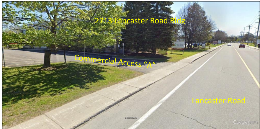
Exhibit 2-5: Lancaster Road / Commercial Access “A” (Looking to the South)
