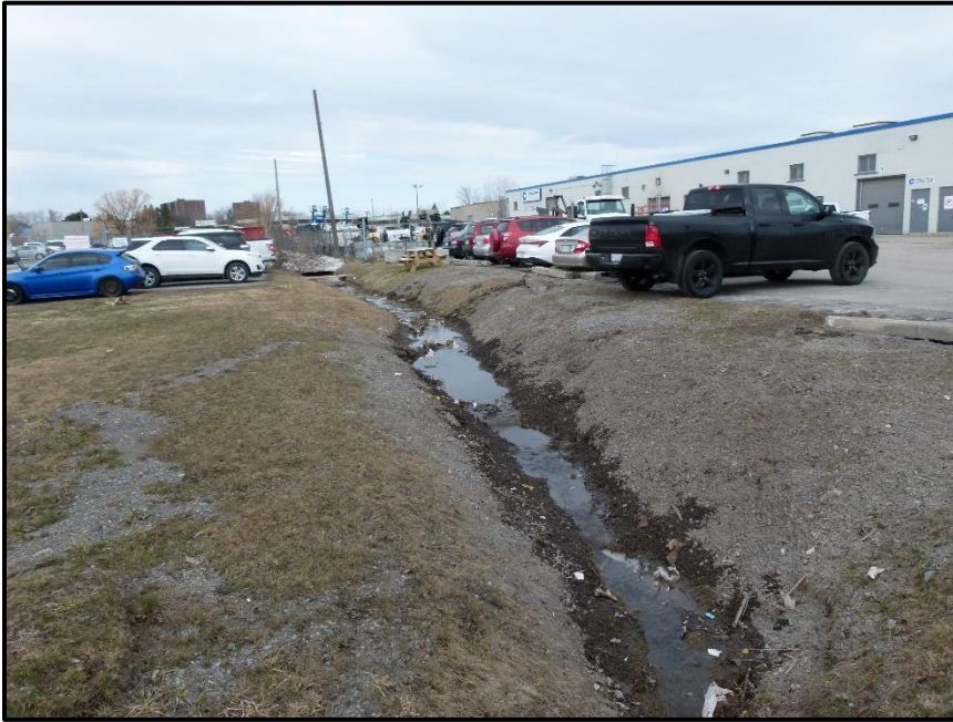
Photograph 3: Looking upstream at the upstream segment of Survey Site #1 (April 12 th , 2023).
