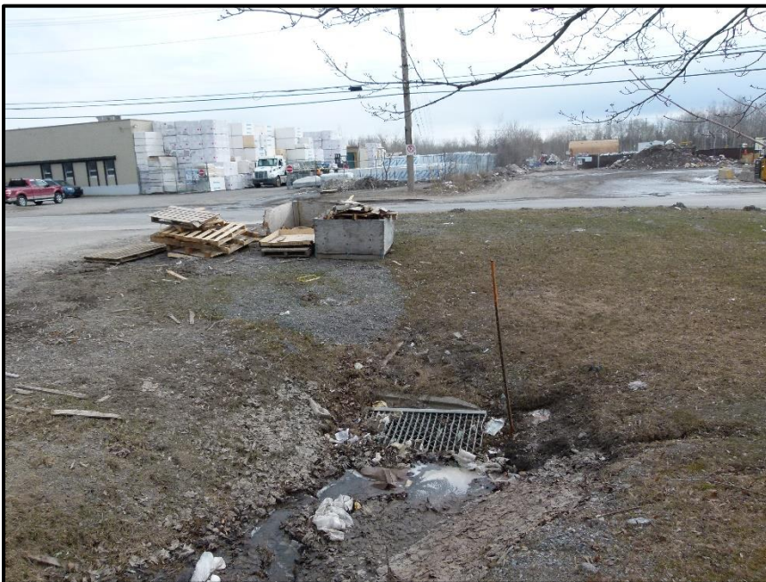
Photograph 2: Looking downstream at the catch basin at Sheffield Road (April 12 th , 2023).
