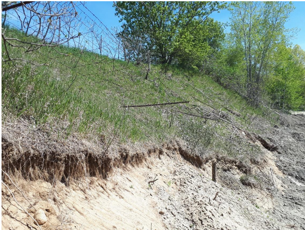
Photograph 11 – View of northwest property line
