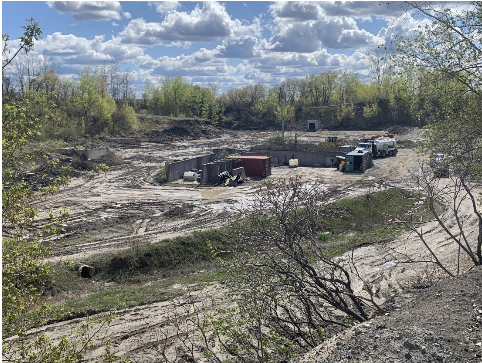
Photograph 1 – Overview of site facing southwest
