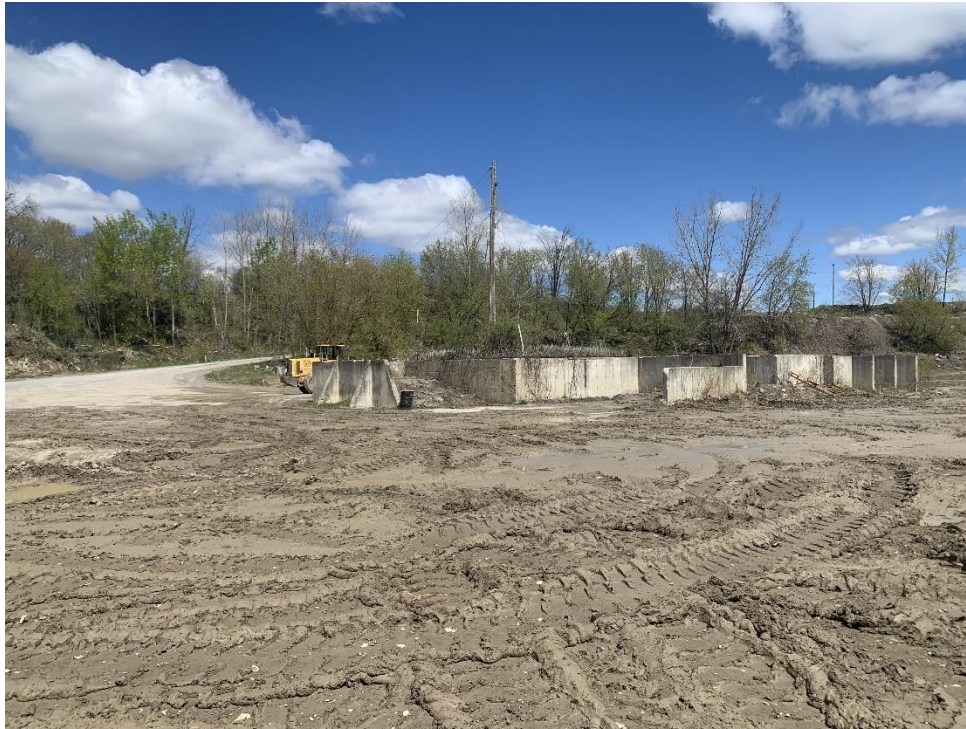
Photograph 3 – View of site facing northeast
