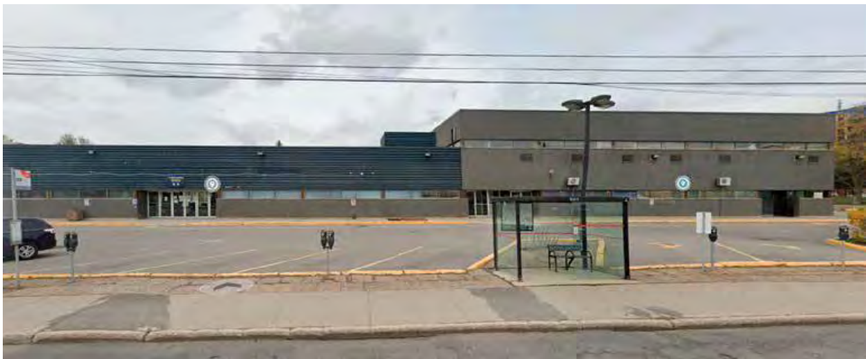
Figure 1 – Former Ottawa Bus Depot (Catherine Street Elevation)
