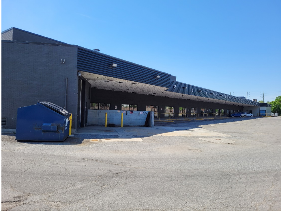
Photograph 3: View of the north side of the Phase One Property looking west. View shows the terminals for the former central bus station. The diesel underground storage tank and former fueling area is visible in this photograph.
