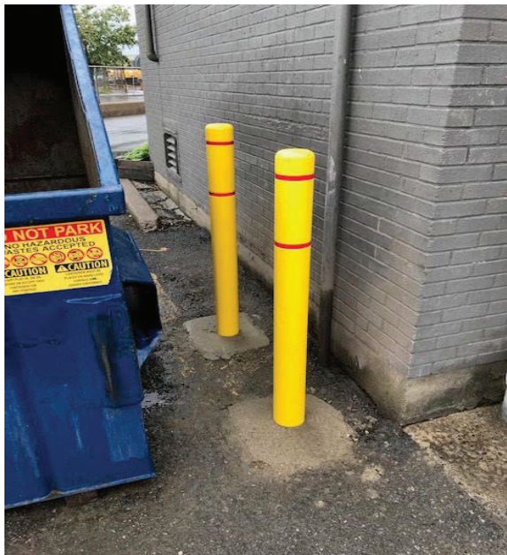
VENT AREA AFTER INSTALLATION OF BOLLARDS
