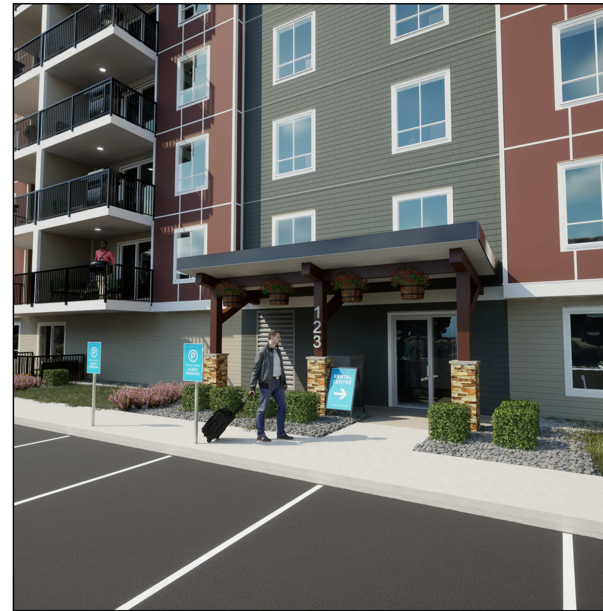
(2) BUILDING A - PRINCIPAL ENTRANCE
