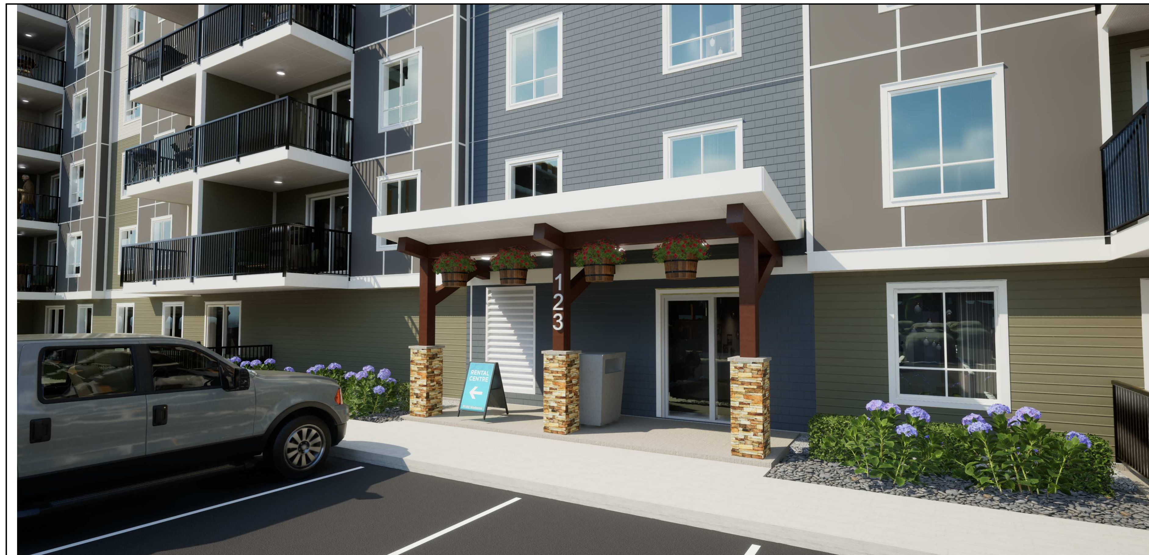
(3) BUILDING C - PRINCIPAL ENTRANCE
