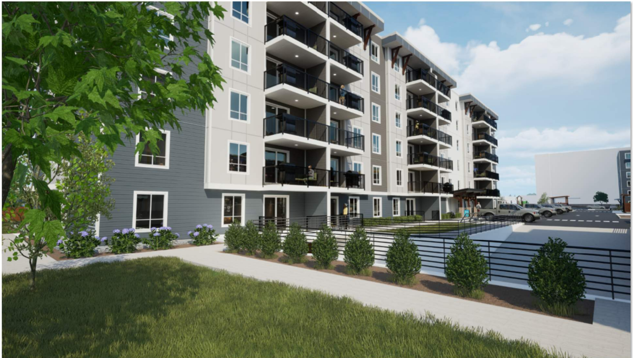
Figure 12: Building D looking northwest
