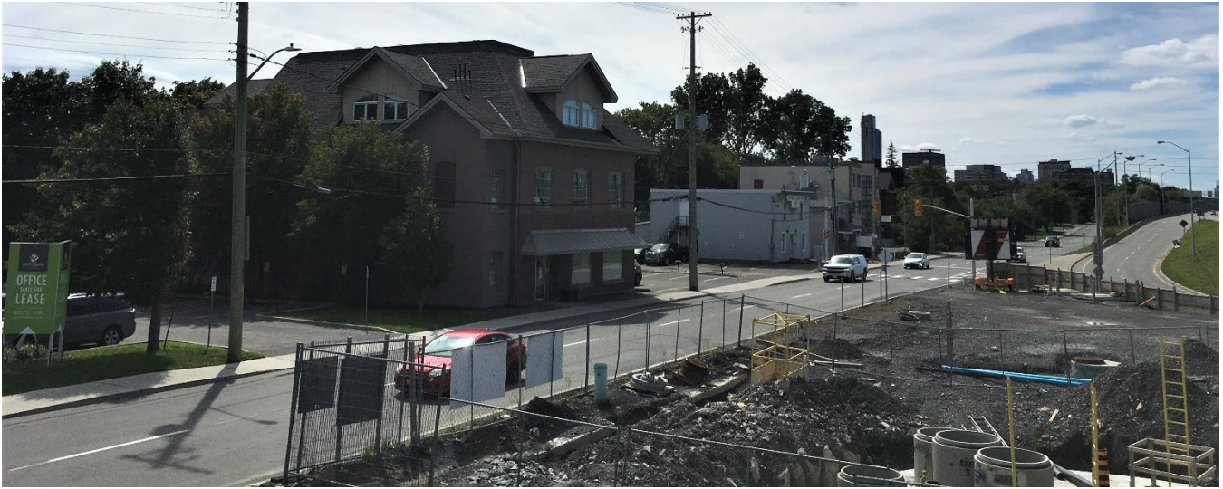
Figure 3: Subject Property looking southwest (existing buildings to be demolished).
