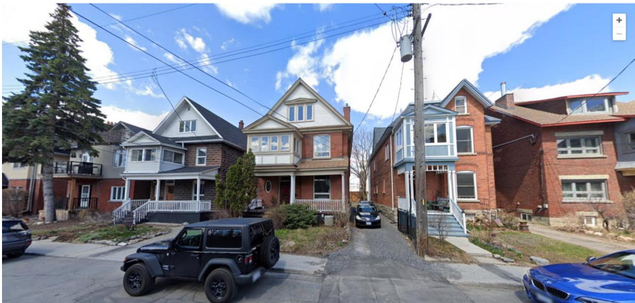
Figure 4: A View of the two 'Registered' properties at 39 and 43 Rosebery Avenue. Neighbouring buildings include the fine example of Boyd Block at 55. An enclosed second-storey balcony with pediment on all three buildings is a common feature along the street where views into Central Park are a focus. Google Earth
