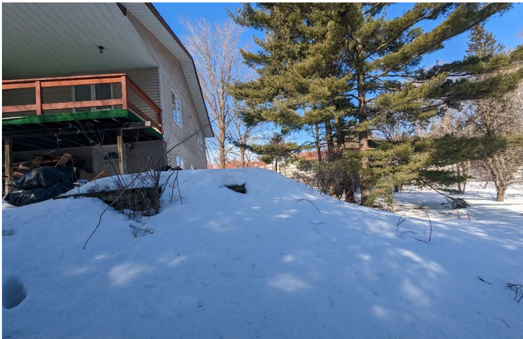
Photograph 4: Rear of building, looking west. Construction debris visible below the deck.
