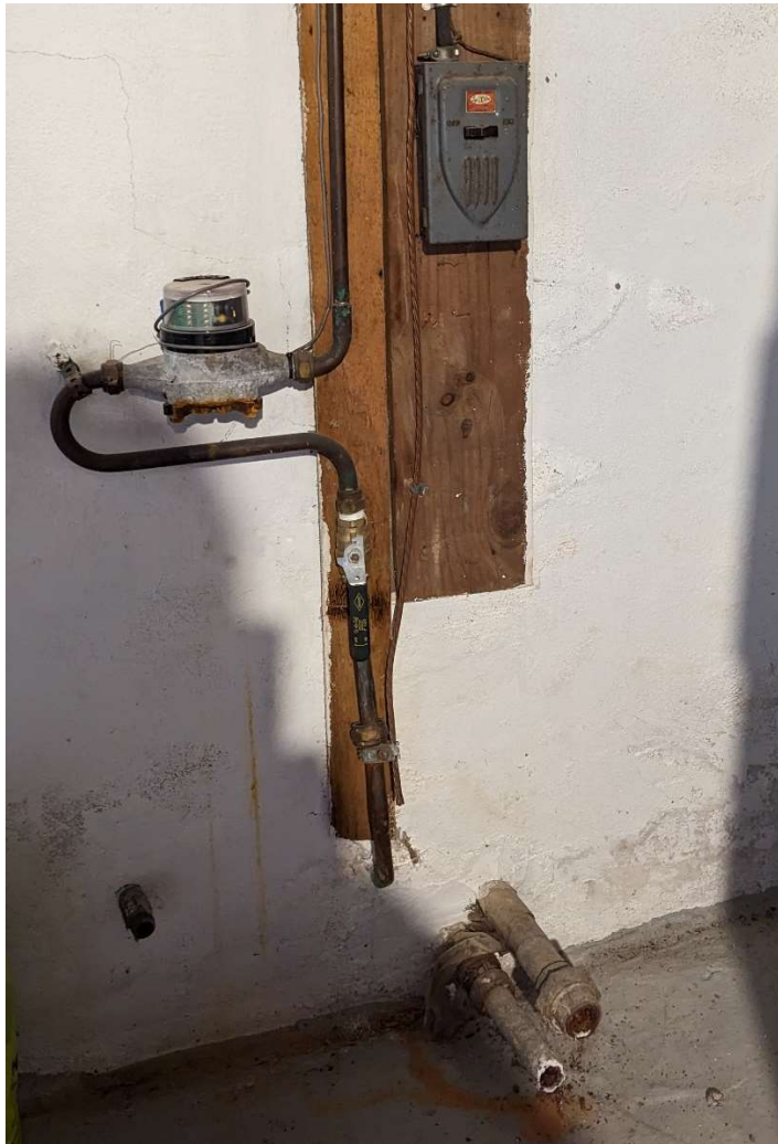
Photograph 5: Original pipes and water meter in basement.
