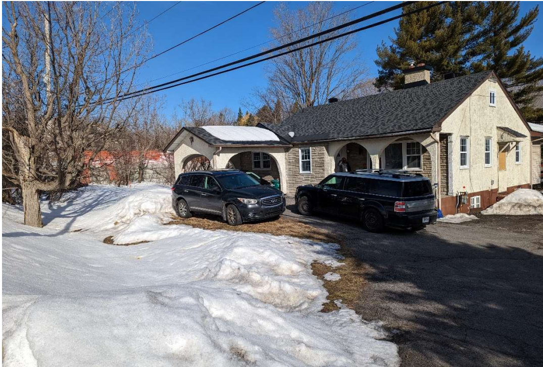
Photograph 1: View of 1815 Montreal Road from the roadway, looking northwest.
