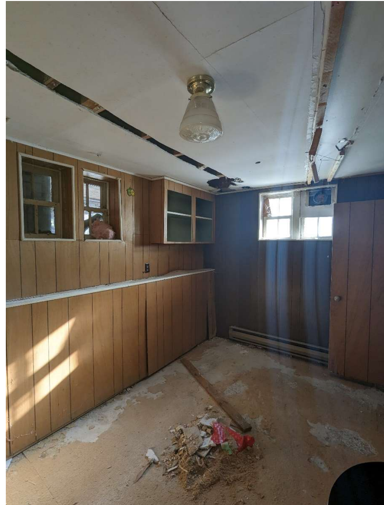
Photograph 6: Unrenovated room in basement.
