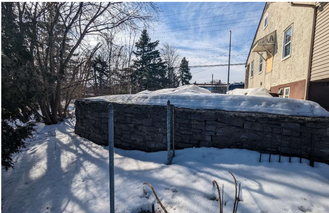
Photograph 2: View of retaining wall north of former private garage, looking south.
