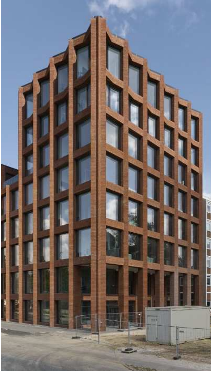
DRAEGERWERK AG, ADMINISTRATION BUILDING, ARCHITECT MAX DUDLER, LUEBECK, SCHLESWIG-HOLSTEIN, GERMANY
