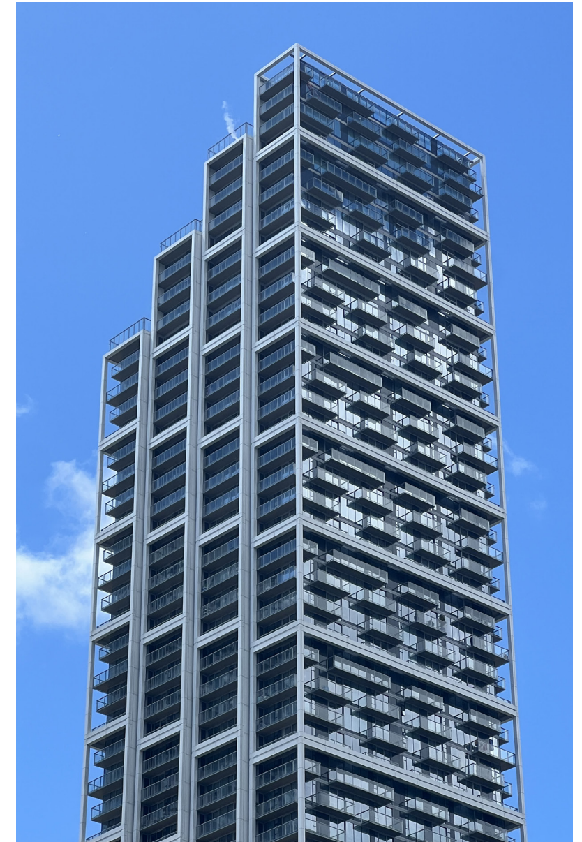
6000 MCKAY AVENUE, BURNABY, BRITISH COLUMBIA, CANADA
