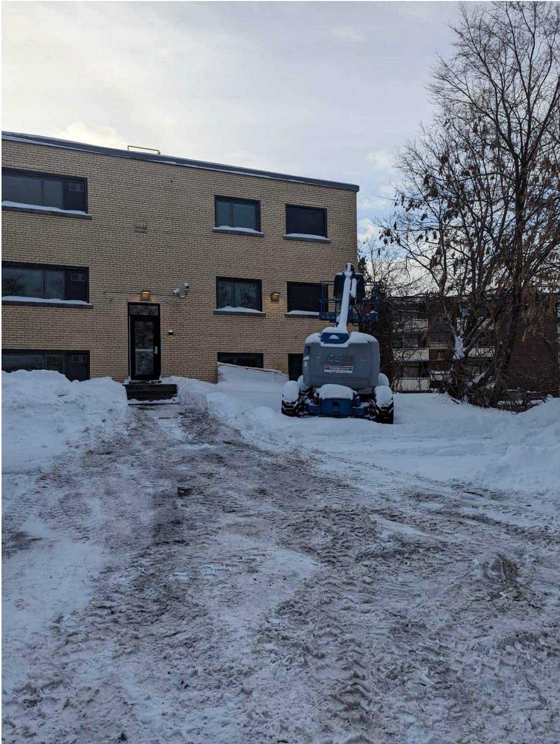
Photo 1: Overview of the exterior of 1095 Merivale Road.
