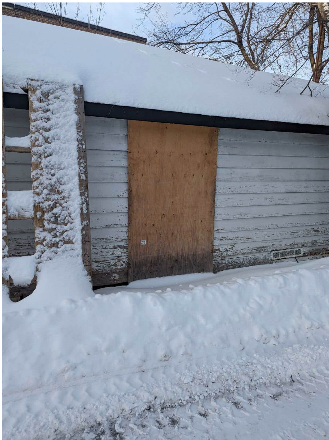
Photo 6: View of the shed north of 1083 Merivale Road.
