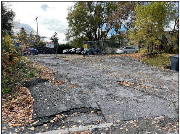
Figure 2-12: Existing access to 1095 Merivale from Panet Street / Emperor Drive, looking south.
