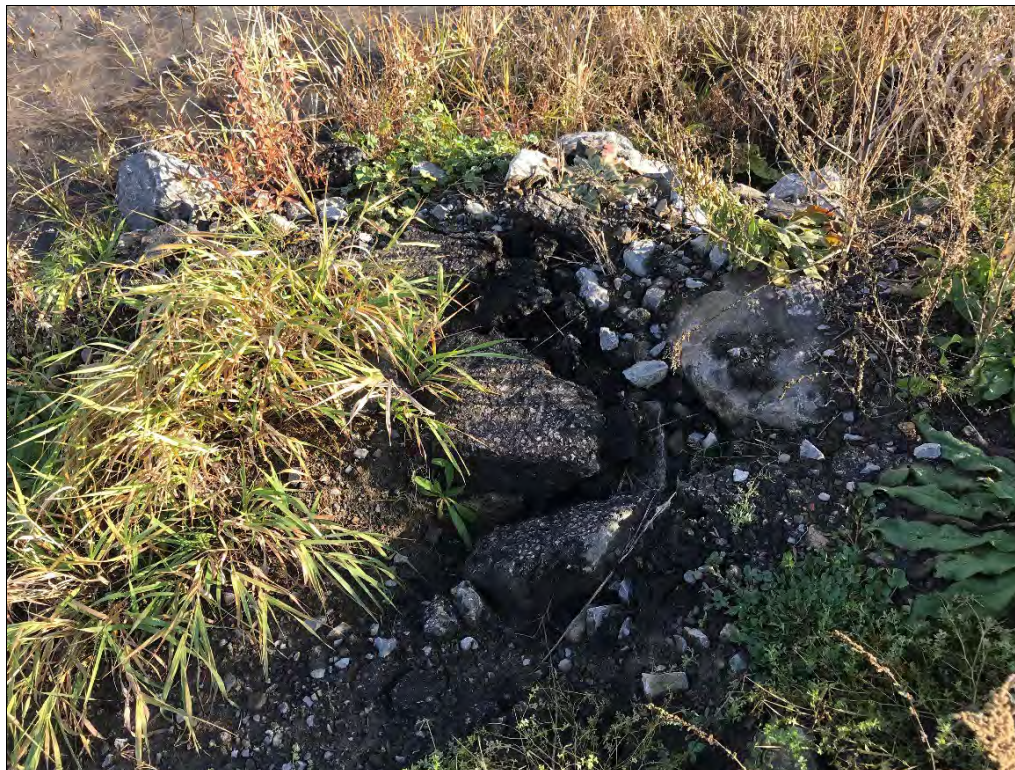
Photo 8: Waste asphalt near the end of the roadway on the western portion of Site. Date: 12/11/21 Direction: N/A
