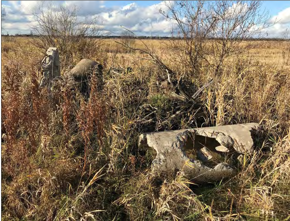
Photo 5: Waste concrete and rebar on northwestern portion of the Site.
