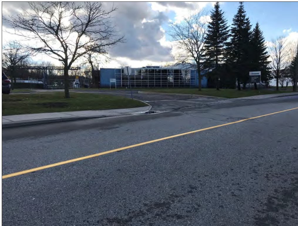
Photo 18: Enbridge and Canada Post facilities to the southwest of the Site Date: 12/11/21 Direction: Southwest
