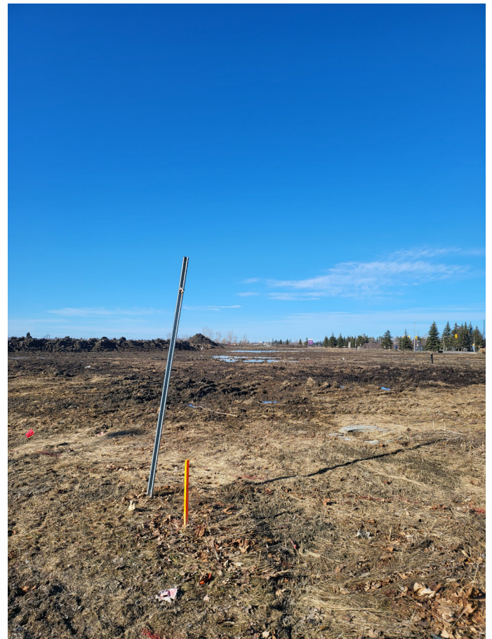
Photo #2 – Looking towards the northeast from the southwest corner of the site.
