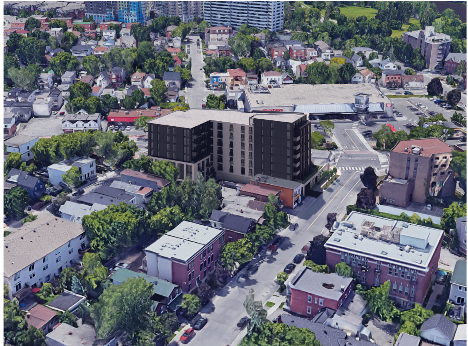
View Looking South
