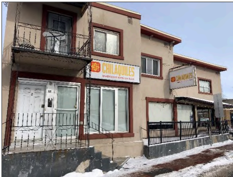
Photo 10 – South elevation of Site Building D, looking northeast.
