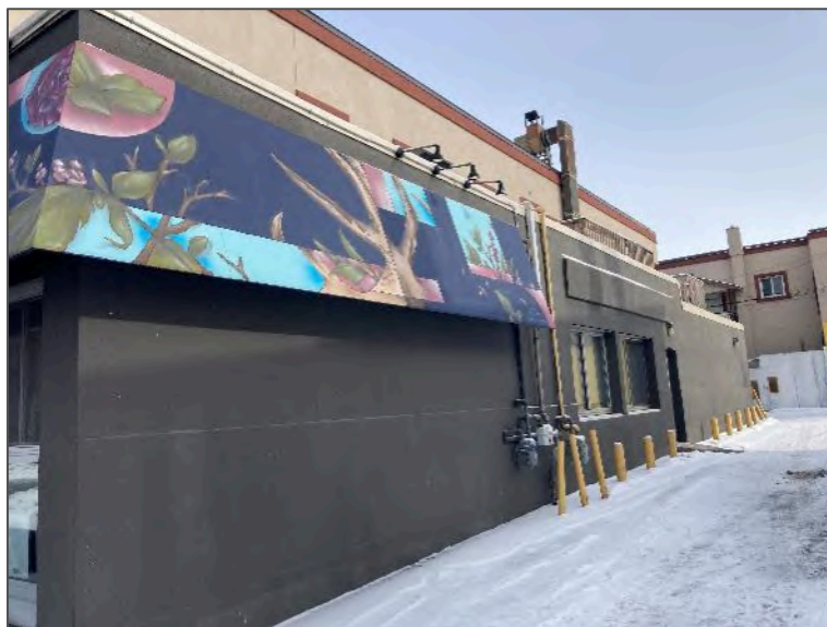
Photo 2 – South elevation of the Site Building A, looking northeast.
