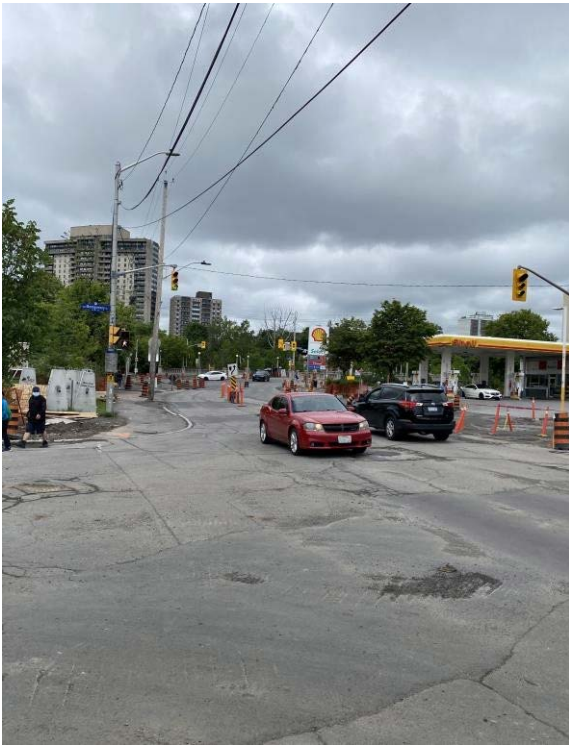
Figure 5: Montreal Road (road reconstruction)
