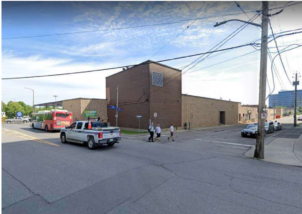
South-West Corner of Property – Facing North-East
