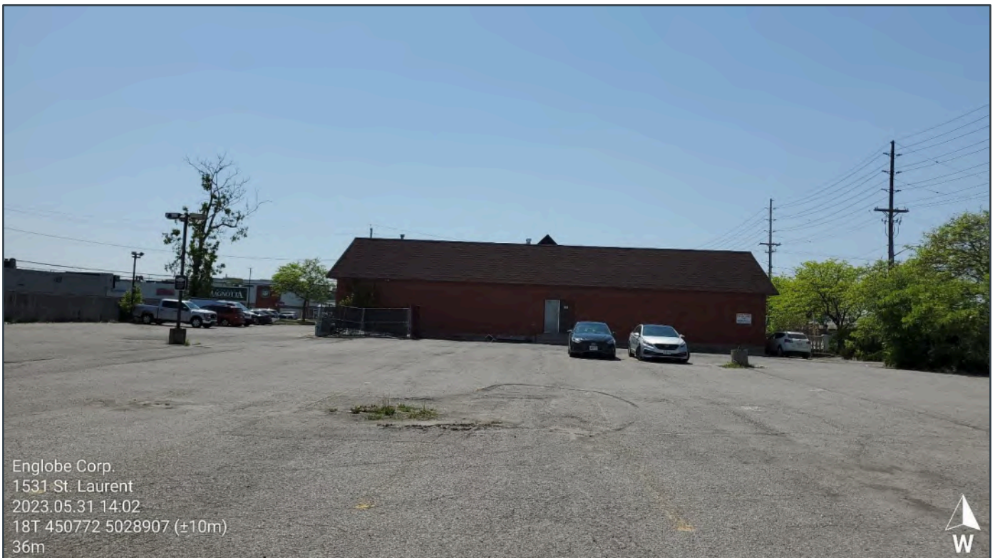
Site Photograph 2: Overview of the rear of the building.
