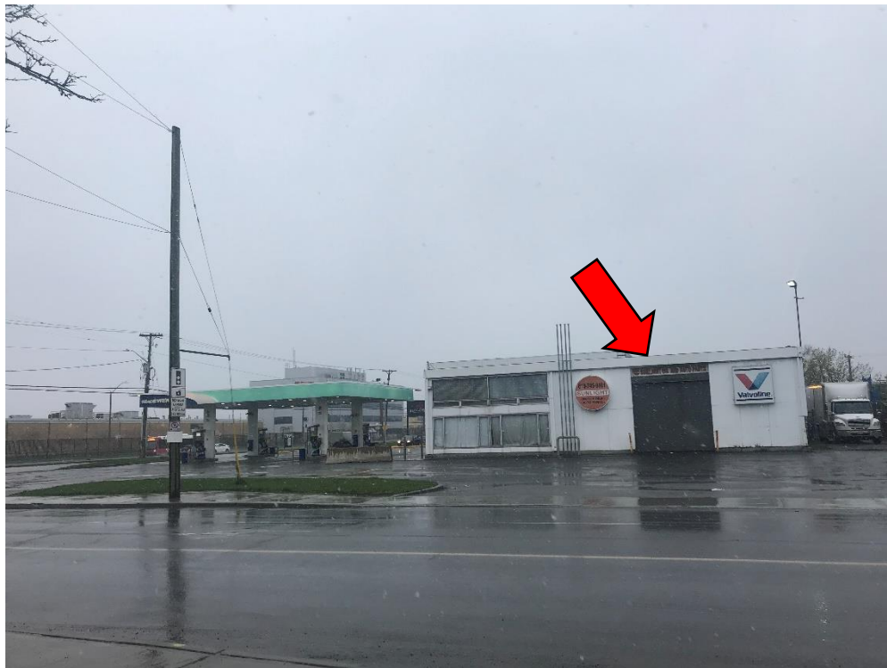
Photo 6: Automotive service garage, located to the north of the Site.
