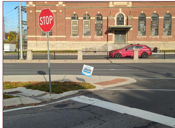
Photograph 8: Power station at 1275 Carling Avenue
