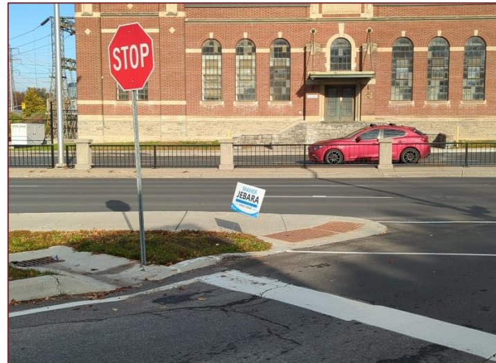
Photograph 8: Power station at 1275 Carling Avenue
