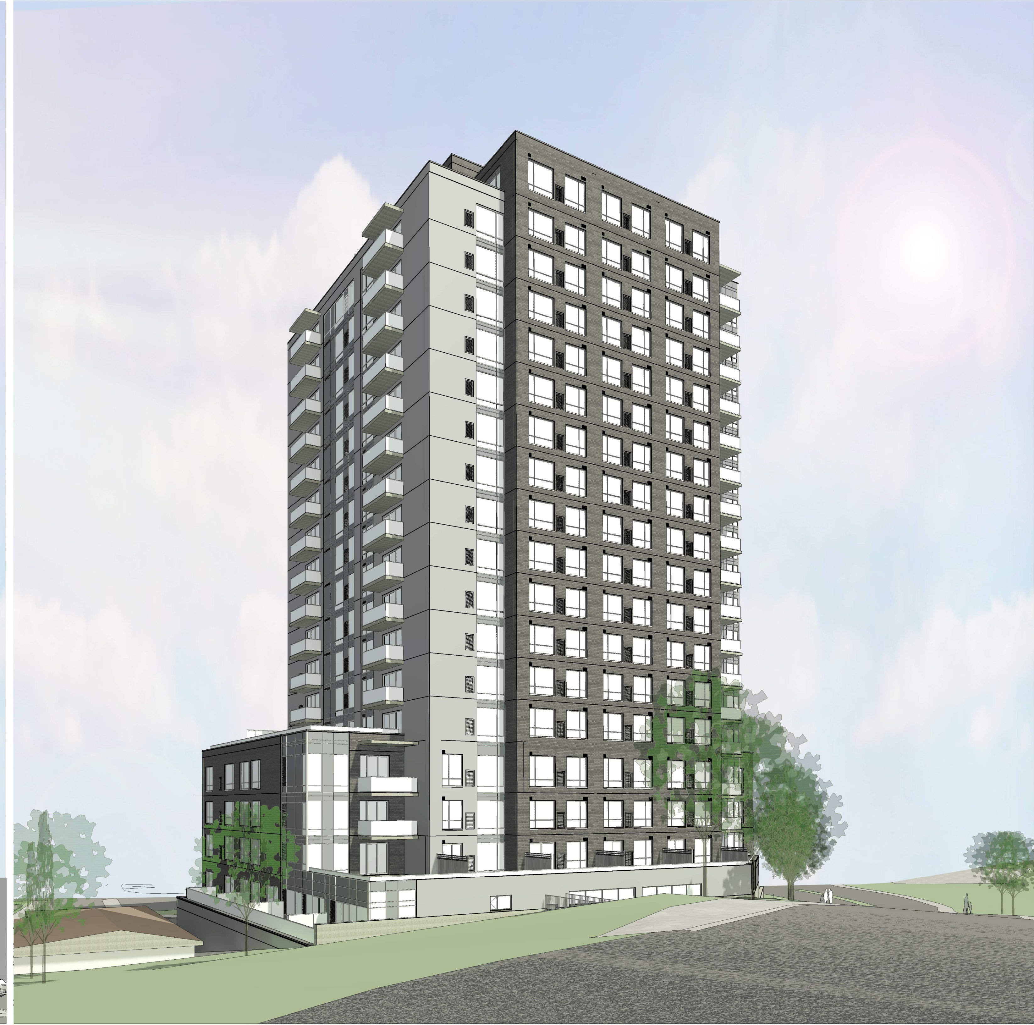
VIEW LOOKING NORTH EAST FROM DUFORD DRIVE
